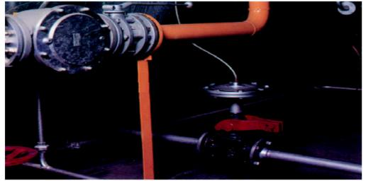
The combination of the Continuous desalting valve\* and the Blowdown valve for bleeding dirt and sludge\* is essential for optimizing the boiler's efficiency, and include its maximum security and availability.
